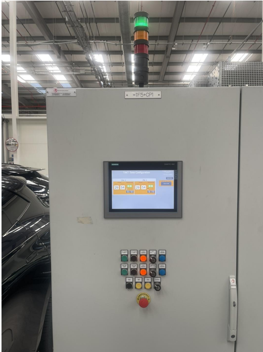
Figure 15-HMI at Aston Martin Lagondas production facility (Purnell-Whitehead, 2025)
