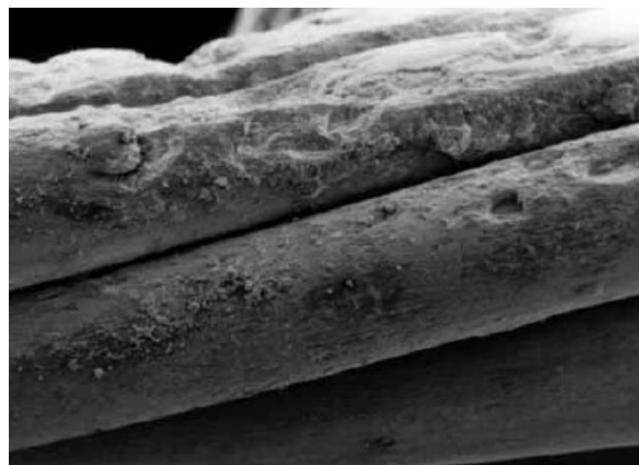
Figure 17 - Pitting on individual wires due to loss of galvanic protection [20]
