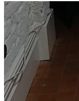
Figure 1 Wire is blue tacked to the wall to take away the risk of a trip hazard
