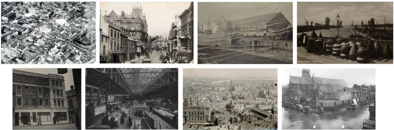
Fig 1 - Swansea Pre Blitz Photos (Swansea Council, n.d.) –
