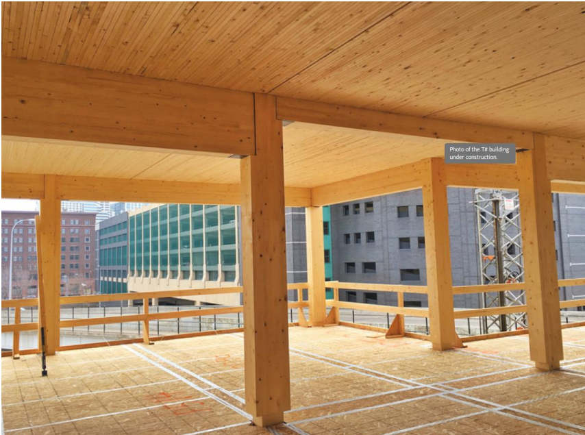
Image 2 Post & beam glulam timber frame structure with CLT and timber floor panels
