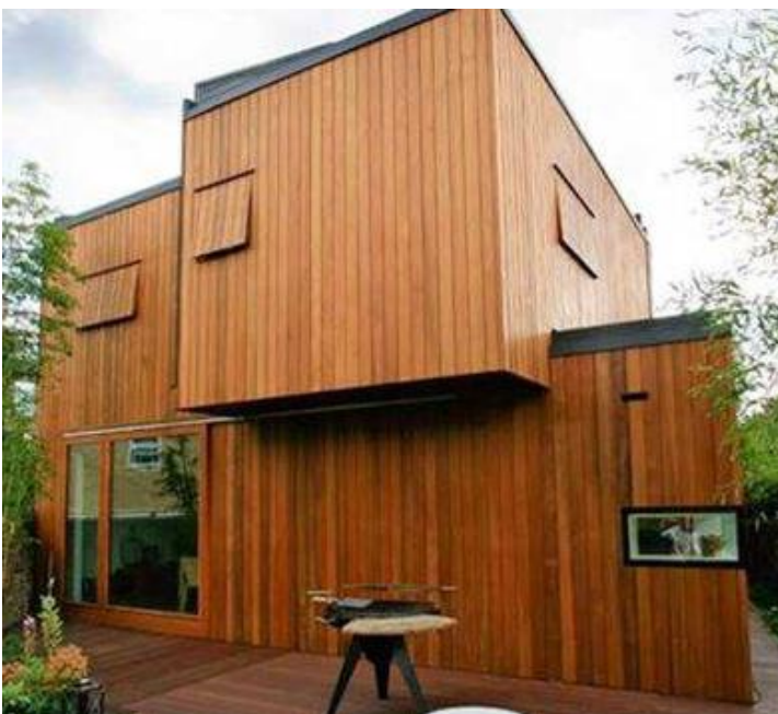
Image 5 Western Red Cedar cladding finish (Latham James The Natural Choice, 2024)
