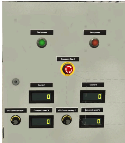
Figure 35 - The Control Panel (Factory IO)
