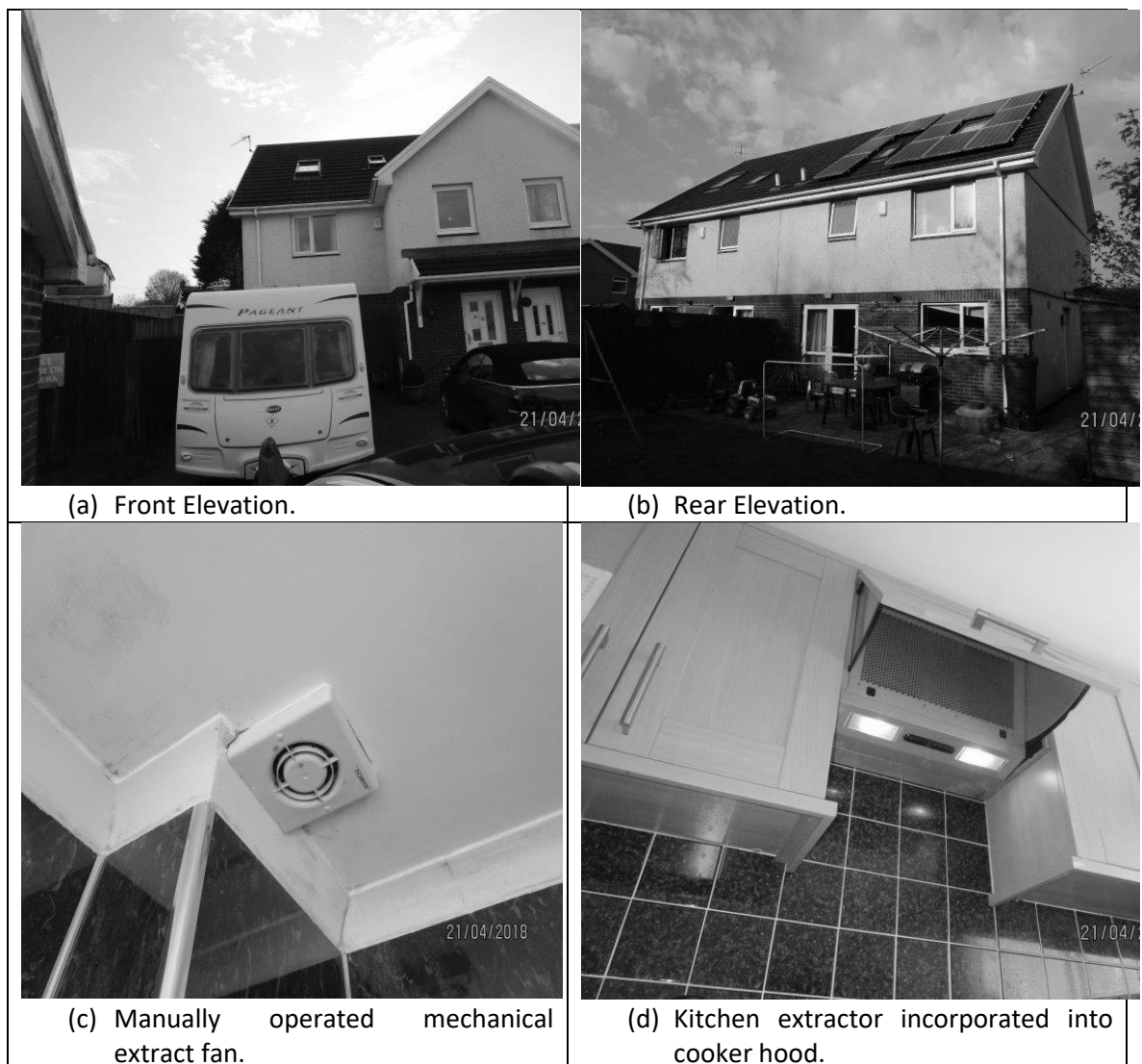
Figure 4.1. 1: Semi-detached 4 bed dwelling constructed 2006 (Francis, 2018).
