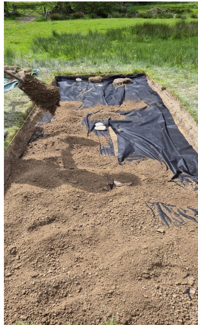
Top right- Filling the trench back up
