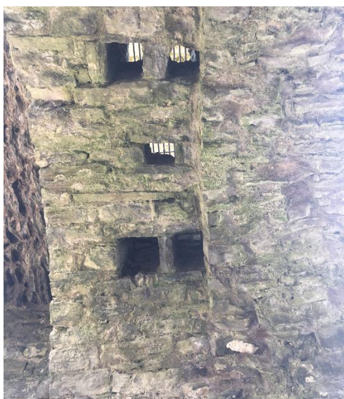
Figure 4 – Murder Holes on the ceiling of the second entrance
