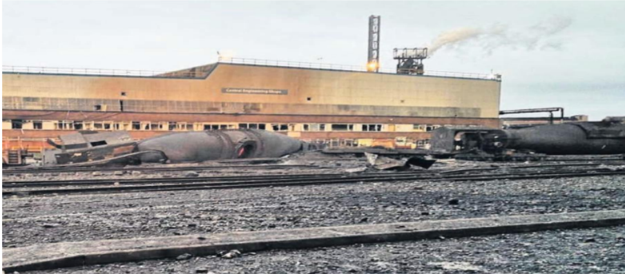
Torpedo explosion in front of Central engineering Workshops (fig 4)
