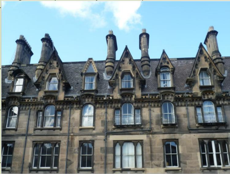
image shows "Victorian architecture in Spital Street" (Traynor, 2011)
