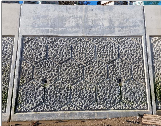
Figure 3 Image of the Mumbles sea wall
