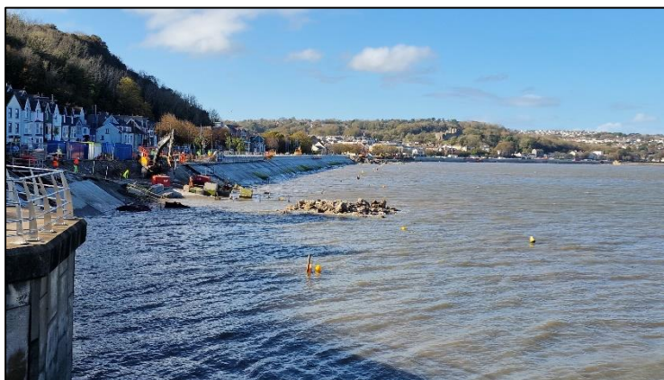
Figure 1 Mumbles sea wall under construction Oct 2024
