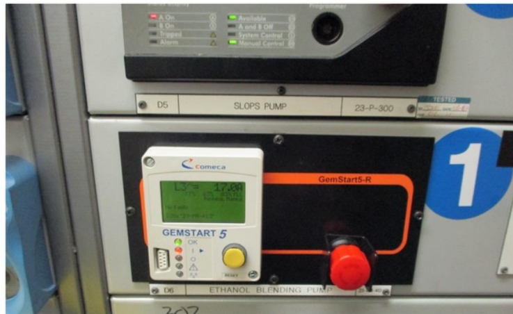
Figure 19 - Motor being ran with coupling installed
