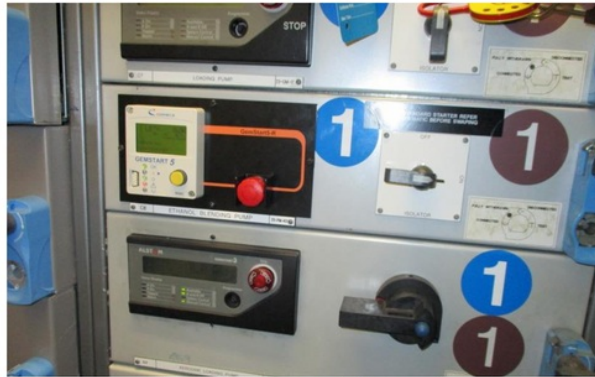
Figure 14 - Starter inserted into carriage
