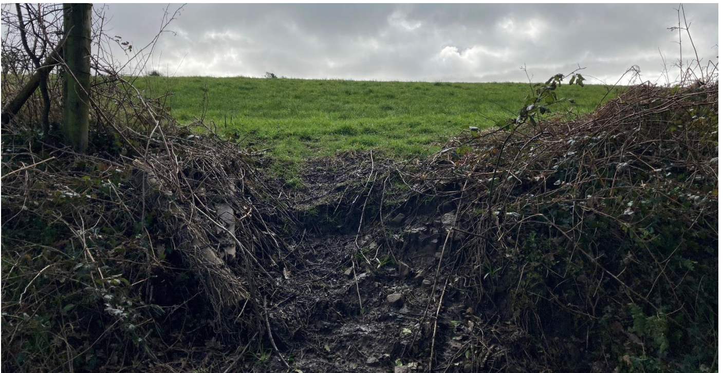
Photo 7: Soil erosion from field run-off
