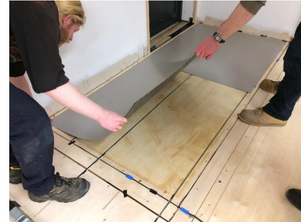
Laying electrical braids and temperature sensors Laying printed metal sheets
