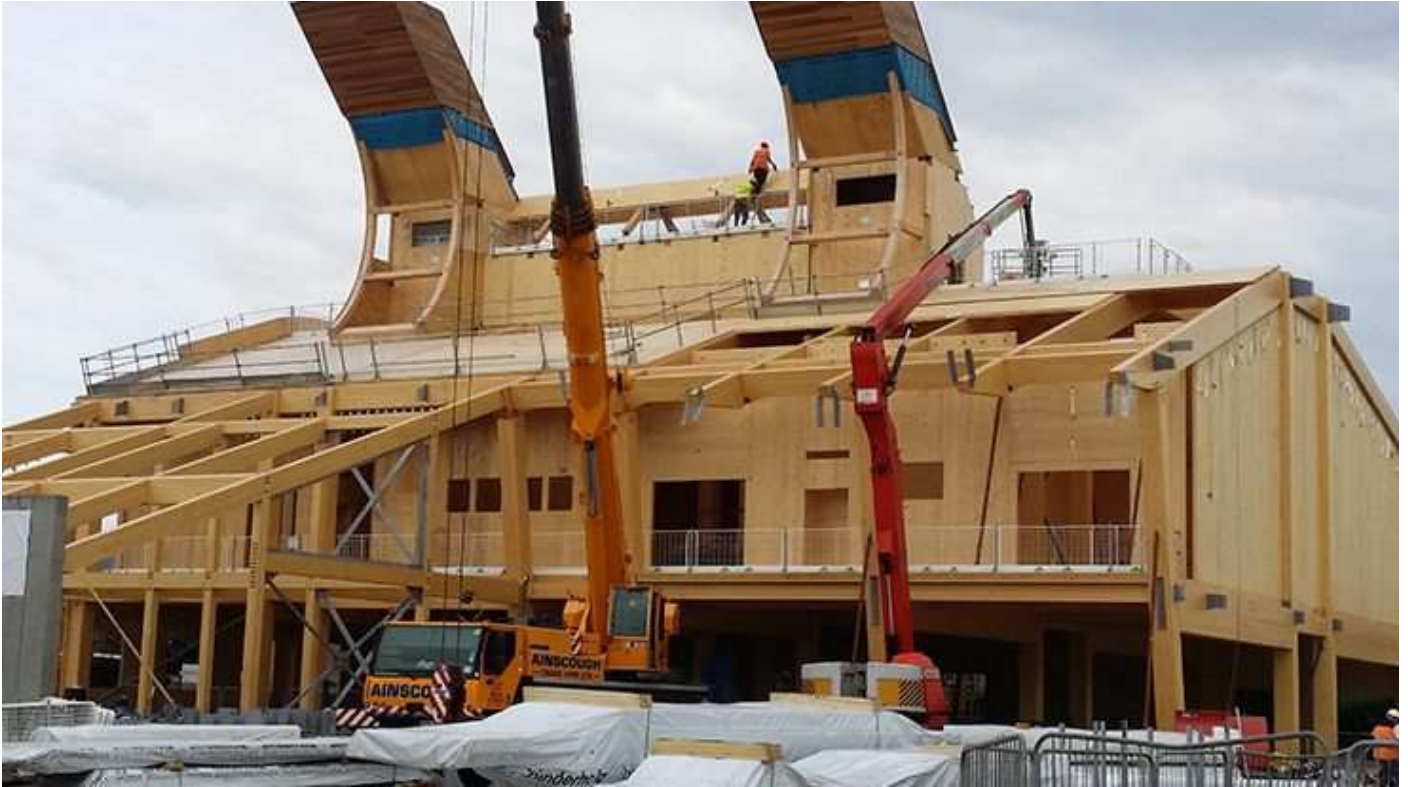
Figure 7 Image above showing the timber structure (Robru Steel Erection, n.d)
