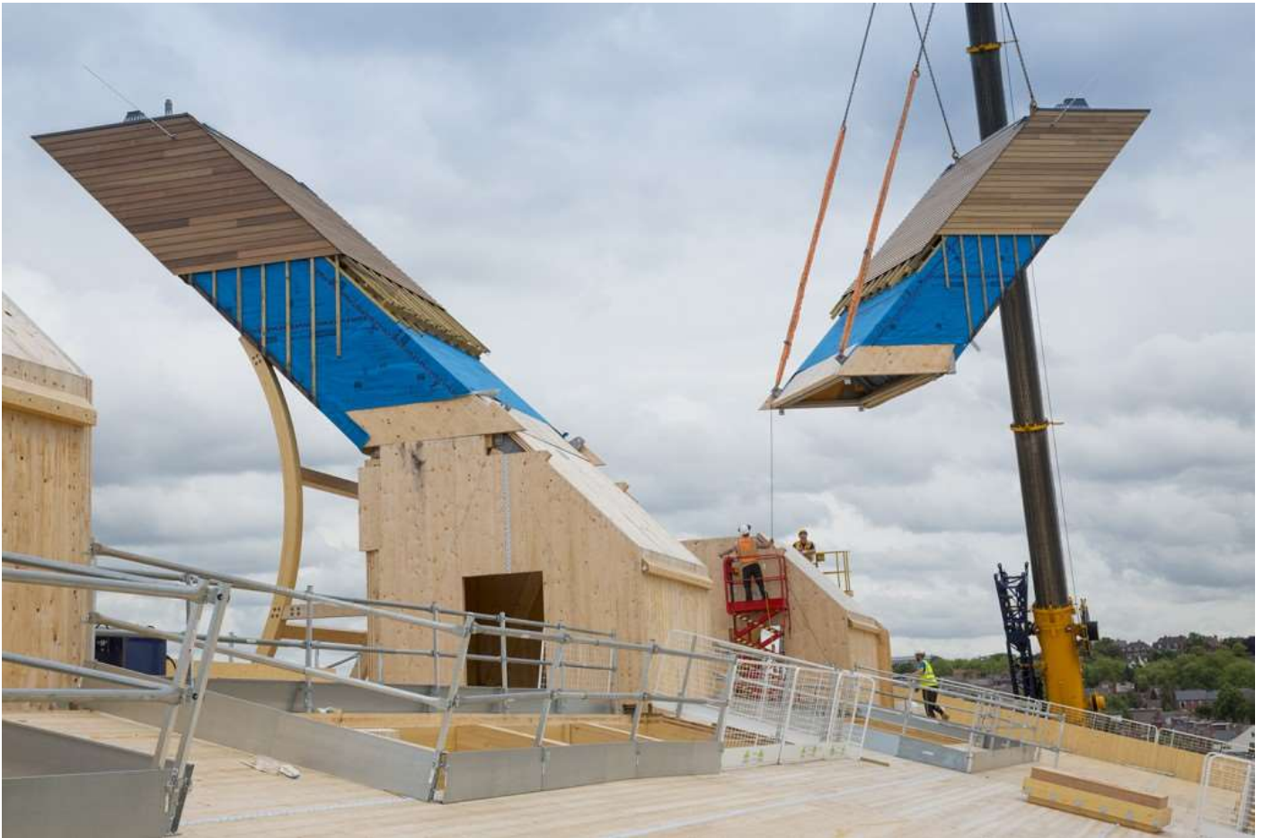
Figure 9 GSK Carbon Neutral Laboratory for Sustainable Chemistry craning ventilation towers into position. (Lowry, 2015)
