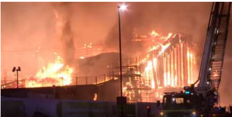
Figure 11 Carbon Neutral Laboratory Nottingham Fire September 2014 (The Guardian, 2014)
