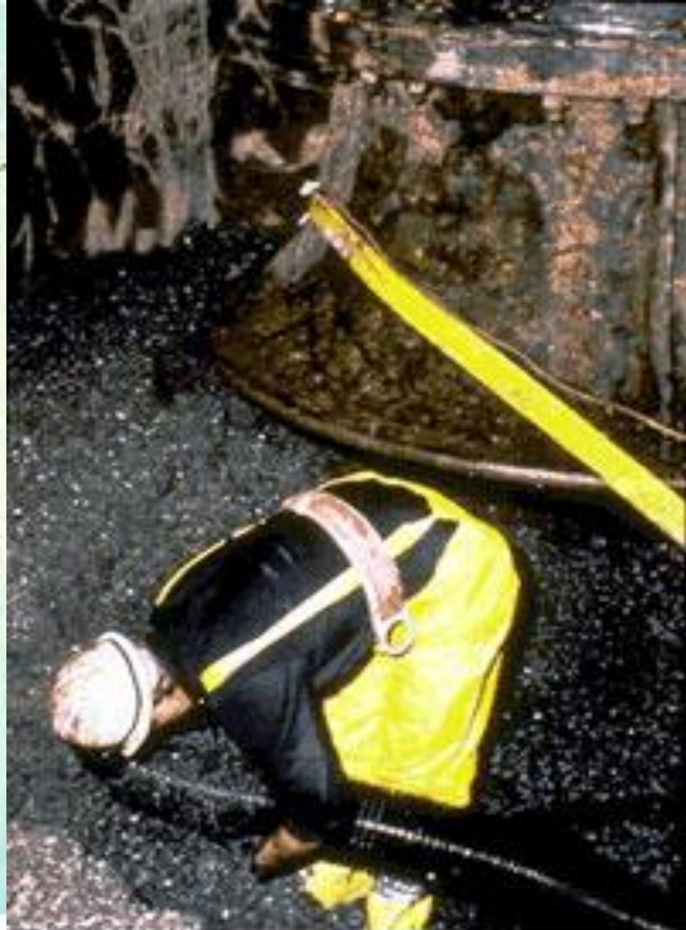
Worker removing zebra mussels from water intake pipes.
