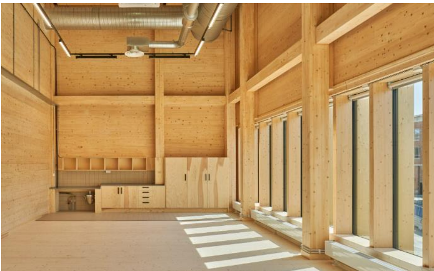
Image 3 Cross laminated timber panels in mass timber structure
