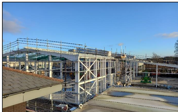
WB Griffith's J604 Pembrokeshire College – Superstructure Steel Frame, including Fall Prevention Railings. Dated 16 th May 2021.
