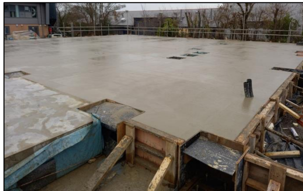
WB Griffith's J604 Pembrokeshire College – Substructure formwork and concrete pour. Dated 22 nd April 2022.
