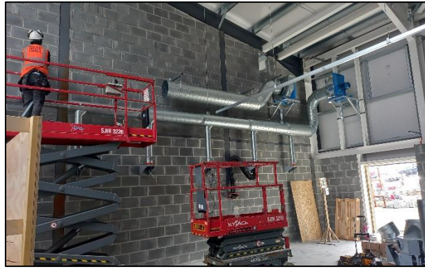
WB Griffith's J604 Pembrokeshire College – Superstructure First Fix M&E Installations. Dated June 21 st 2021.
