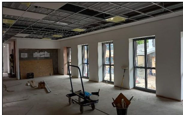
WB Griffith's J604 Pembrokeshire College – Superstructure Drylining. Dated July 5 th 2021.
