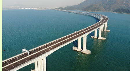
Hong Kong-Zhuhai-Macao Bridge
