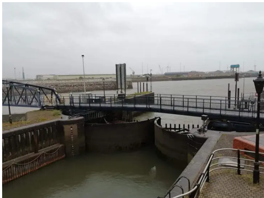
Figure 8: Floodgates Swansea Docks: Swansea Bay News (2022) ‘Storm-damaged marina bridge and lock gates reopen after major investment’ Available from https://swanseabaynews.com/2022/07/07/storm-damaged-marina-bridge-and-lock-gates-reopen-after-major-investment/ [Accessed on 10/12/2022]
