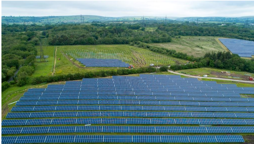
Figure 2: Morriston Hospitals Solar Farm (ITV,2022)
