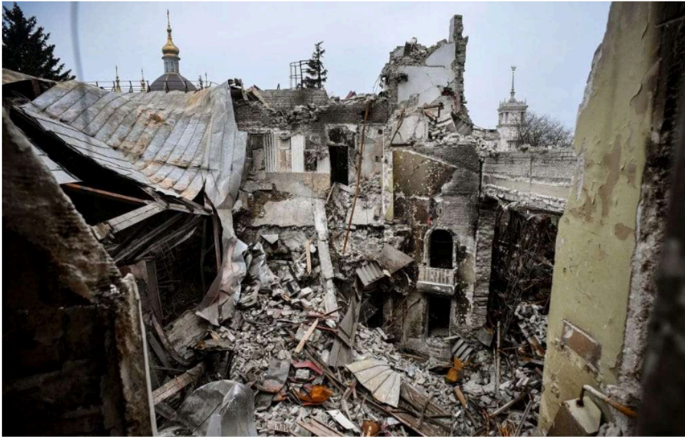
Figure 7 - Mariupol Drama Theatre auditorium after the attack
