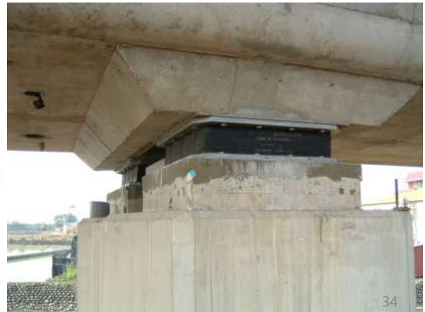
Elastomeric Bearing under combined Compression, Shear & Rotation
