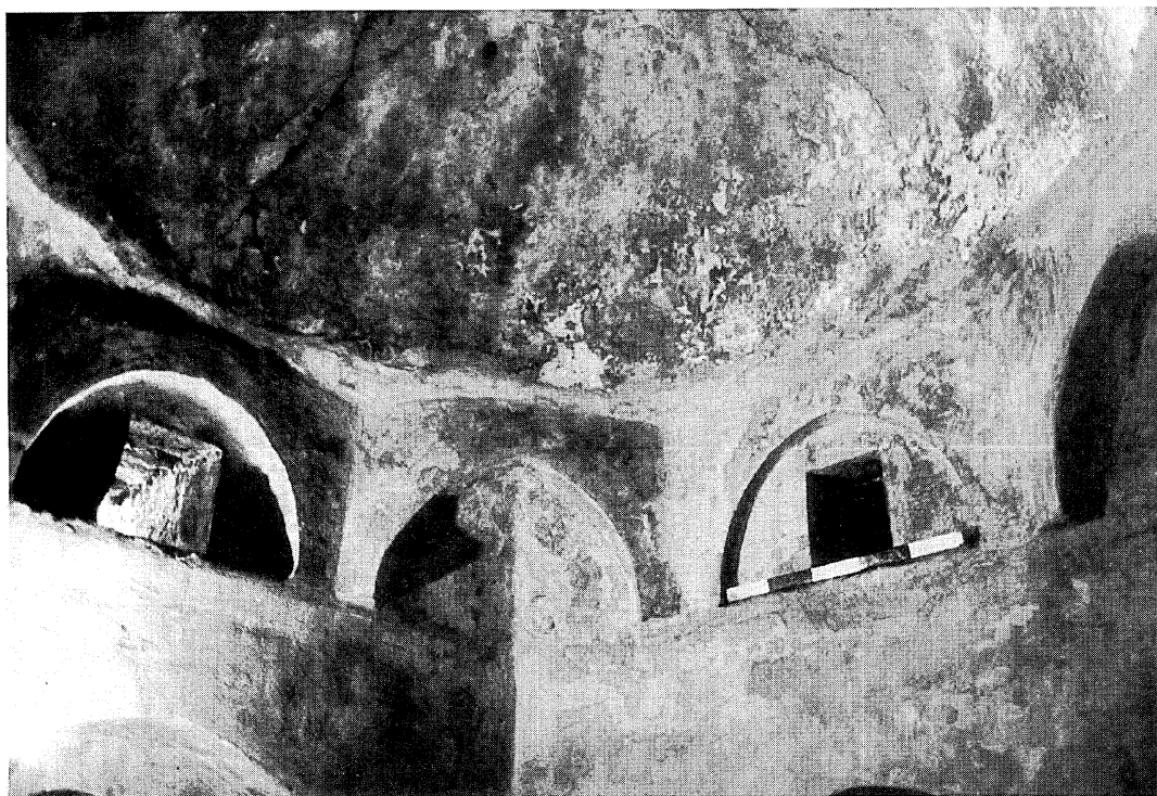
Figure 14. Shaykh Hammar: interior of domed chamber tomb showing corner squinch (MOS no. 73, 2).
