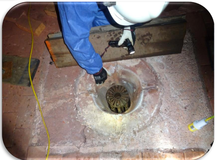
Figure 23: Burner quarl inspection
