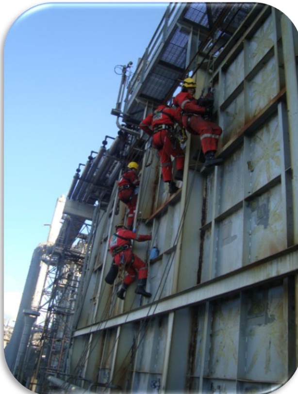
Figure 27: CAN rope access technicians performing inspection of the furnace casing
