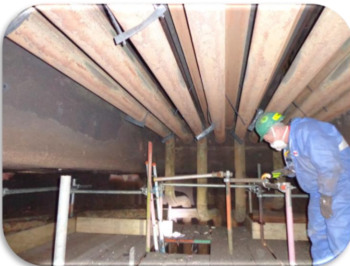
Figure 21: Visual inspection of the roof tubes and radiant sections
