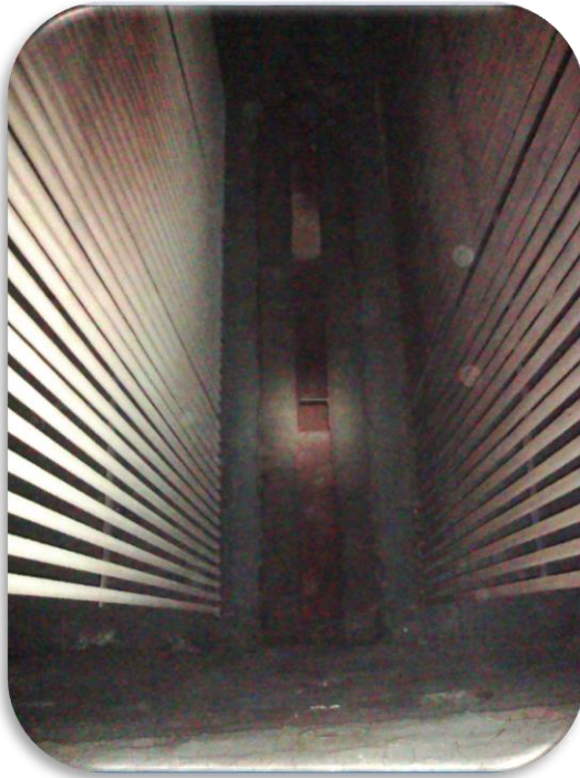
Figure 19: Internal configuration of furnace tubes passes.
