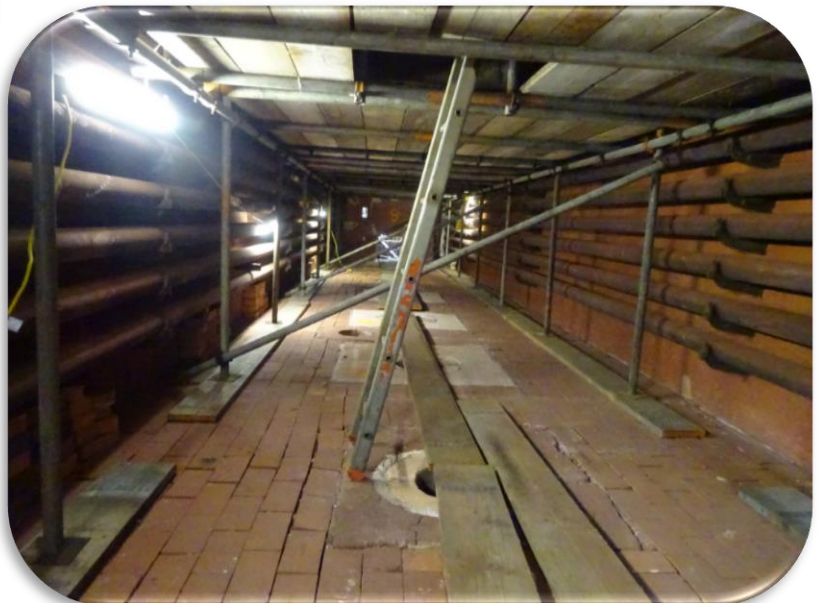
Figure 20: Levels of scaffolding to allow access wall tubes for damage mechanism assessment.
