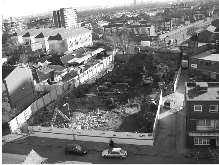
Plate 2 - The excavation works as viewed from the tower of All Saints' Church (photo courtesy of Bugler Developments Ltd.)
