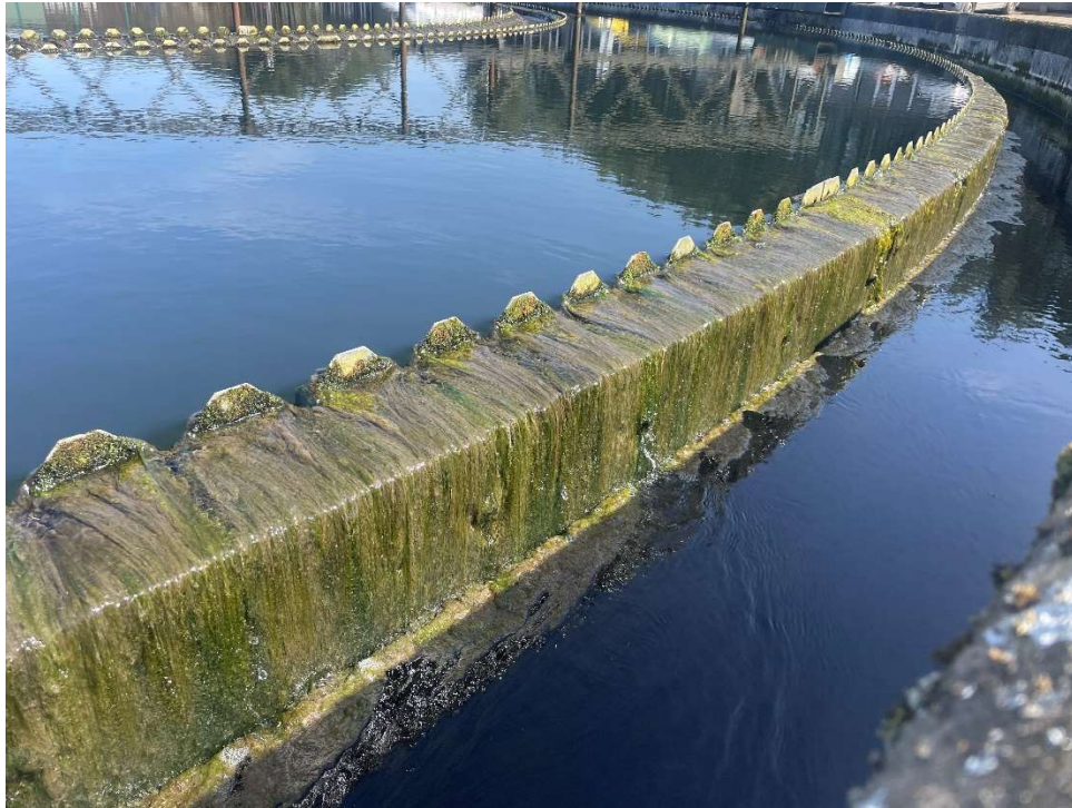
Figure 3 - Primary Settlement - filamentous algae growth.
