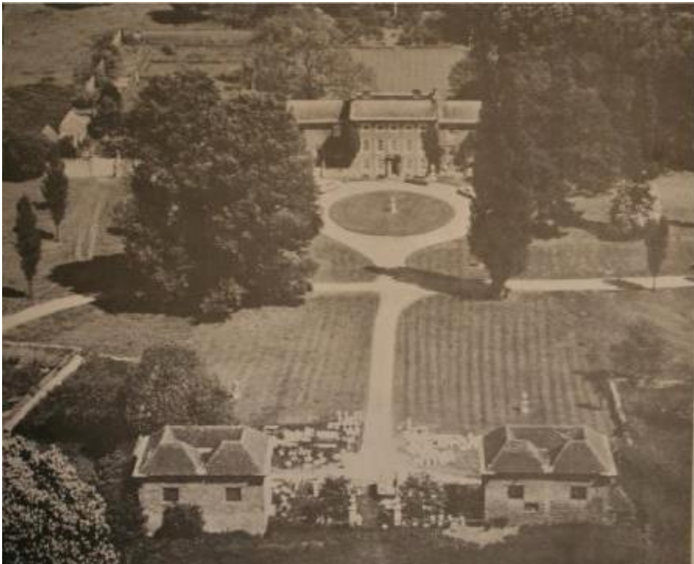
Aerial view of the Manor and Pavilions showing Chilstone ornaments (Andrew Hiorns, 2013)
