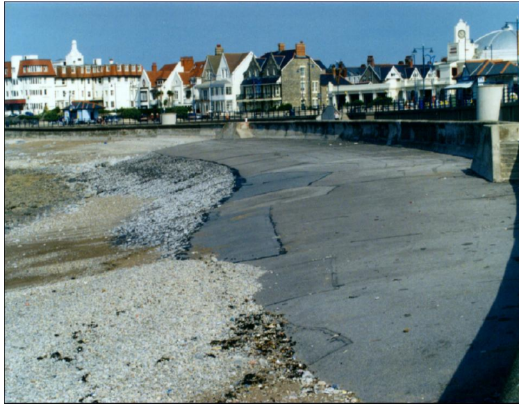
Figure 7: Bitumen revetment
