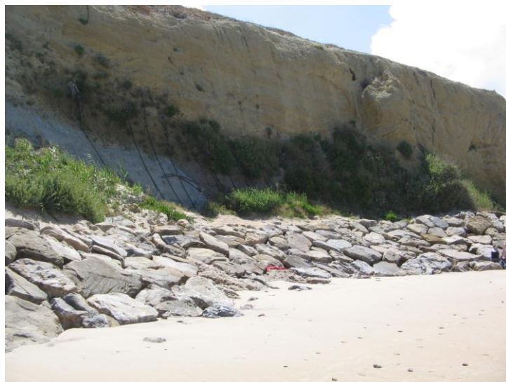
Figure 4: Cliff protection measures
