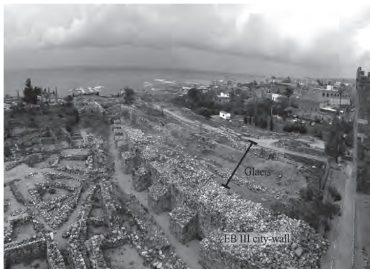
Fig. 1 – Byblos: view of the juxtaposed fortification works on the northern side of the site; in the foreground, the EB III buttressed city-wall; behind it, the juxtaposed glacis dating from the EB III to the Persian Period.
