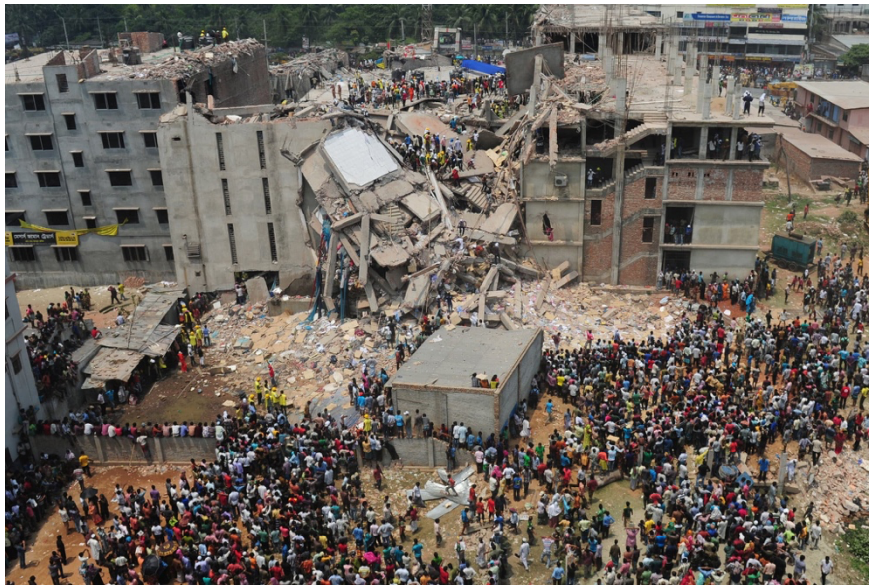
Fig.3 : Rana Plaza building collapse
