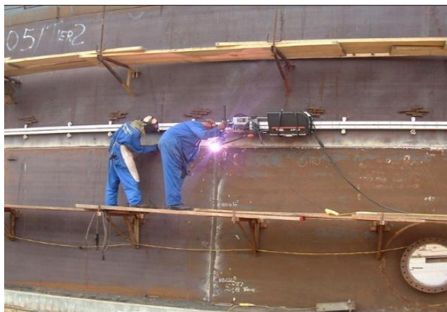
Figure 5 Tank Joint Welding - Oil Storage Tanks (Casagrande Júnior, 2025)
