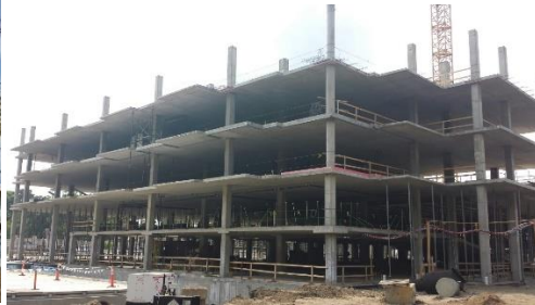
Reinforced Concrete Frame
