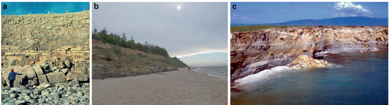
Rock Coasts, Fig. 4 (a) Toppling failure, Glamorgan Heritage Coast, UK (left); (b) Translation on glacial deposits, Poland (center); (c) Rock fall, Sardinia, Italy (right)
