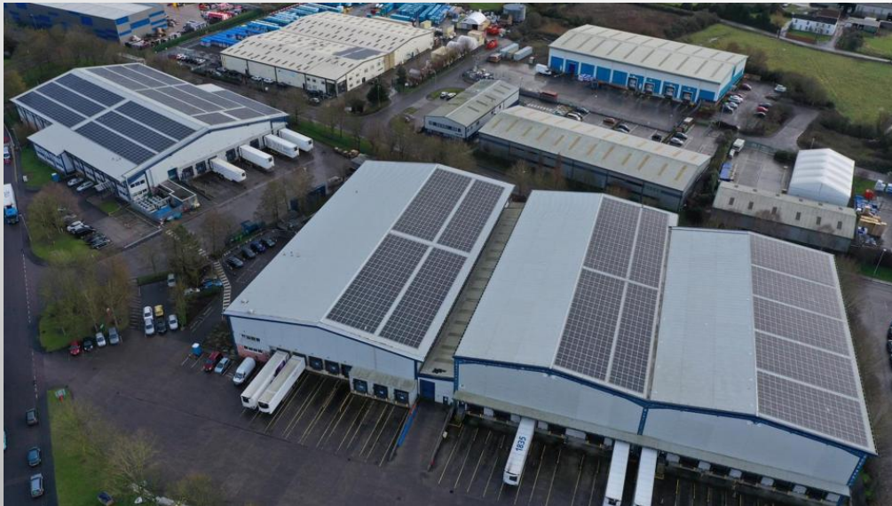
YEO VALLEY SOLAR PANEL
