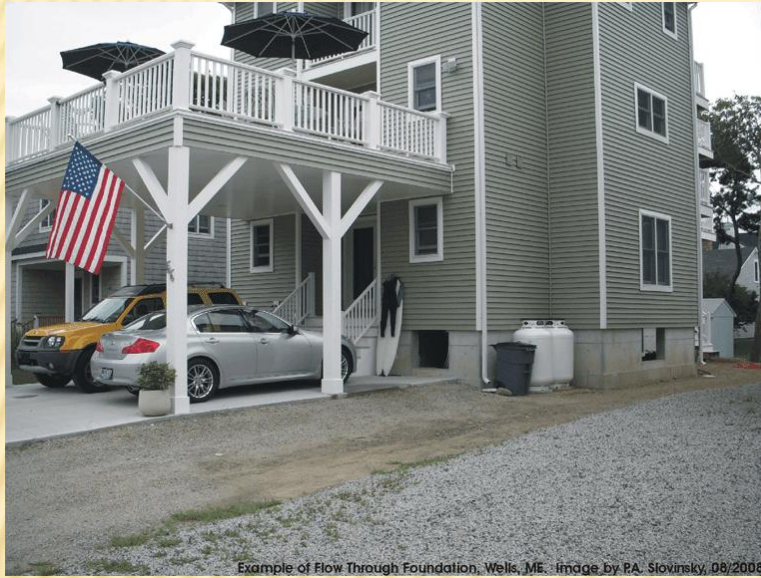
Example of Flow Through Foundation, Wells, ME. Image by PA. Slovinsky, 08/2008.
