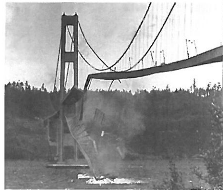
In November 1940, just months after its completion, a large section of the Tacoma Narrows Bridge crashed into Puget Sound in Tacoma, Wash. The bridge collapsed under high winds, a failure that shocked engineers at the time
