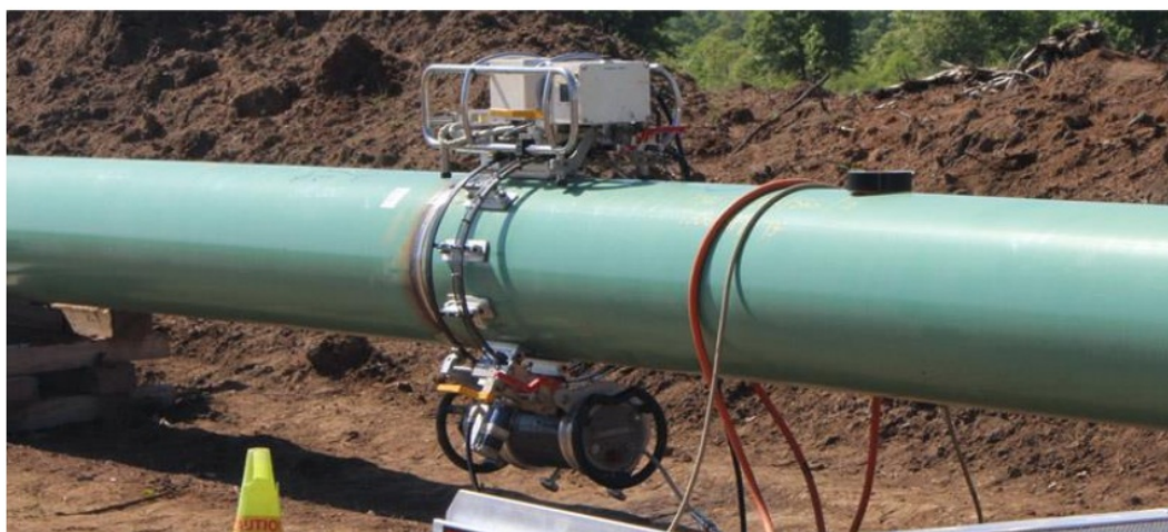
Figure 6: Radiographic equipment scanning a gas pipe (Shawcor, 2019) .
