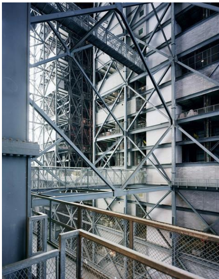
Thomas Struth, Vehicle Assembly Building, Kennedy Space Center , 2008
