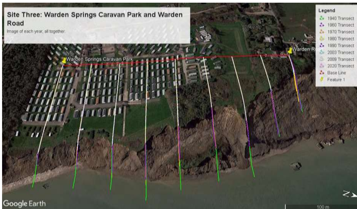
Figure 4.37: Warden Springs Caravan Park to Warden Road with Each Years Transect Lines
