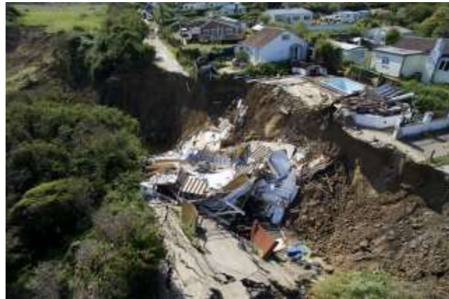
Figure 1.4: The House at Surf Crescent Road over the Cliff, sat on top of the landslide, 2nd of June 2020
