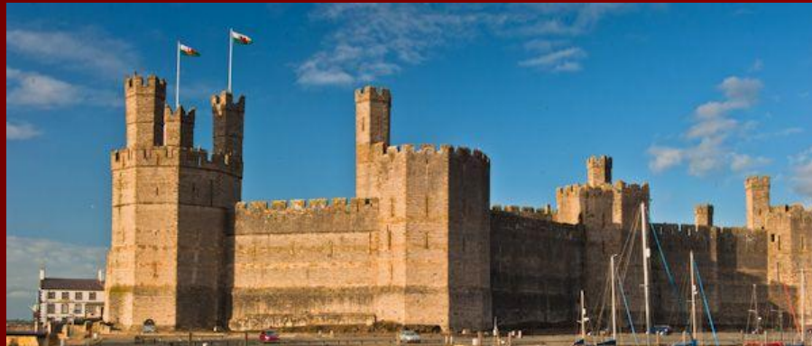
Castles and Town Walls of King Edward in Gwynedd
