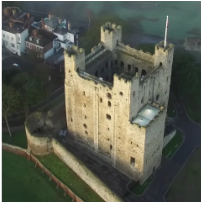
Figure 3: Elevated view of the East drum tower of Rochester Castle, looking West. Henry III's patching can be seen here also. "Drone DJI Phantom 3 Pro – Rochester Castle Kent", Ali-Buck Drone Strike Vids, pub., 2/1/2016, YouTube.
