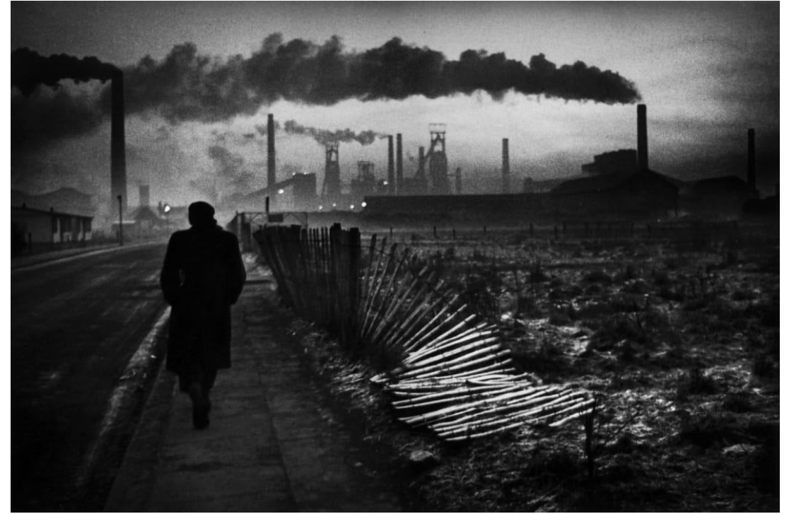
EARLY MORNING, WEST HARTLEPOOL STEEL FOUNDRY, UK, 1963
