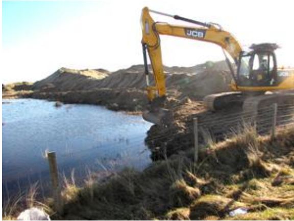
Cleared northern dune side arm behind excavator with temporary platform at its base.
