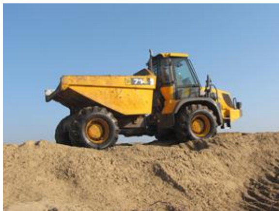
One of two dumper trucks used throughout the contract to move sand and spoil.
