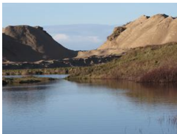
Trough excavation A4 cut into tall foredunes. Flooding in foreground is in area E. Taken about a fortnight after completion on 2 February 2013
