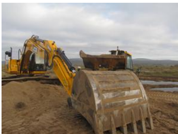
Tracked excavator with digger bucket and dumper truck during trough digging work on 11 January 2013
