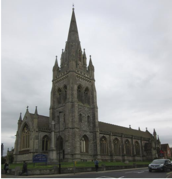
All Saints Church, Queens Road, Ryde Condition: Satisfactory Repair
