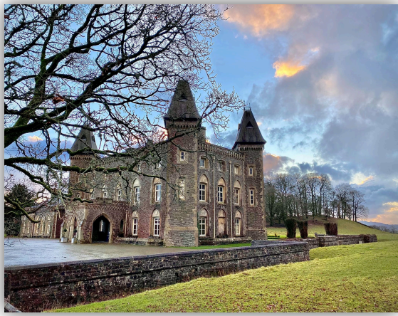
Image showing the turrets, arched windows and lime stone on the north and east elevation. (Author. 2020, Newton House (Photograph))
