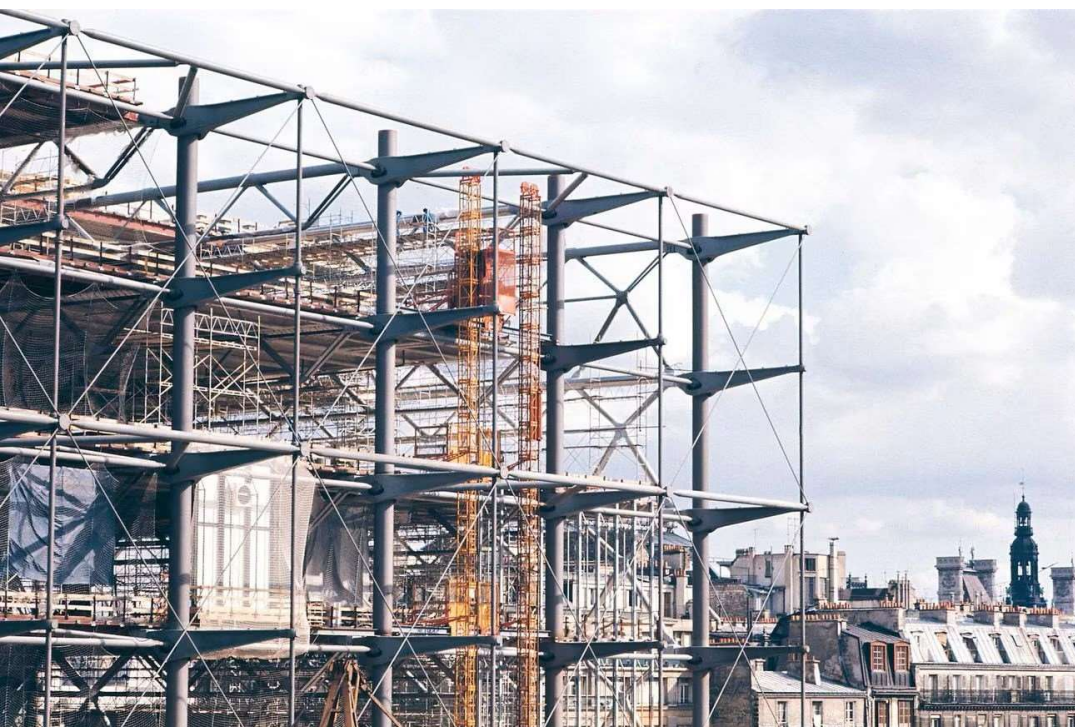
Fig. 7: Centre Pompidou under construction (Vincent, 1975).
