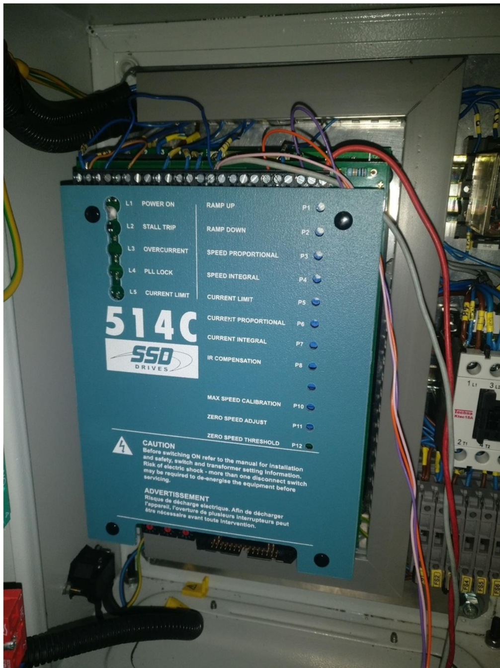
Figure 5.17 – Parker 514C Inside Panel
