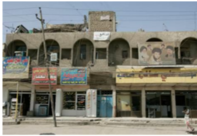
Figure 2: Building in Baghdad [4]
